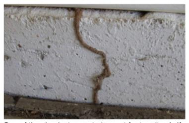
One of the simplest ways to inspect for termites is if you have an unfinished basement. Look around for "mud tubes", that climb up from the base of floor. These tubes protect the termites as they come to the surface, as they don't like sunlight. These tubes are formed from a gritty sand-like substance.
