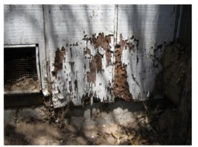
Exterior structures, where the wood is consistently unprotected from the weather, tends to retain moisture in the wood panels. This is typically less dense wood, again being perfect conditions for termites to invade.
