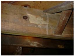
Wood beams in the basement can have visible damage at times. If you feel "soft" or hear "hollow" wood once you tap on it, that's a sign.
